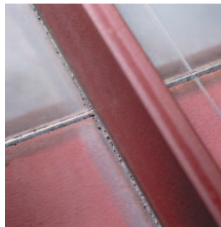
Butt and fillet joint
